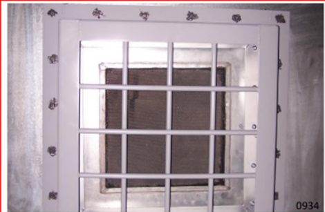
Supply Air Ceiling Penetration; RF Vent & Security Bars
