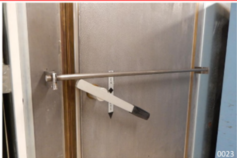
Entry Door – Steel Bar & Brackets
