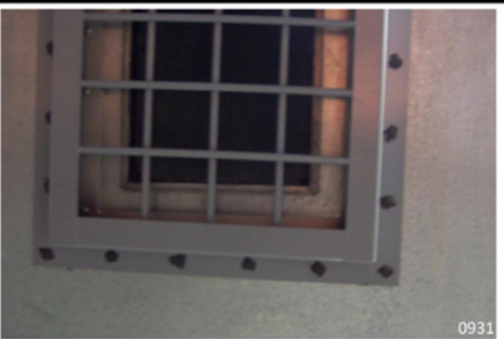
Return Air Ceiling Penetration; RF Vent & Security Bars
