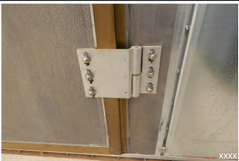
Entry Door – Bottom Hinge Epoxied
